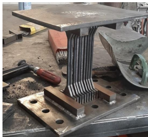
Figure 4. Prepared yielding damper to be installed in the concrete moment-resisting frame
