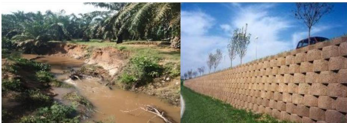
Figure 2: (a) River Cliff Shape at Research Location (b) Segmental retaining wall reinforced with segmental elements with geosynthetic reinforcement.
