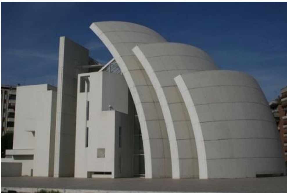
Figure 1. Jubilee Church, Rome, Italy. In the facade of this structure, concrete with a combination of titanium dioxide nanoparticles has been used [3].
